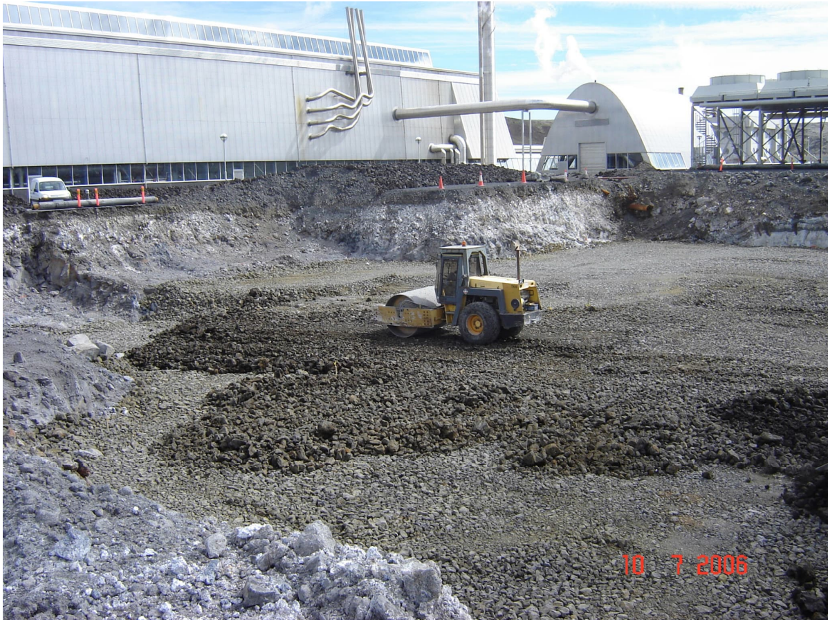
Figure 3.3 Earthwork for power station 6 in July 2006.
