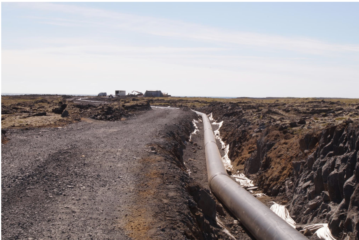
Figure 3.2 Installation of pipeline to Arfadalsvík.
