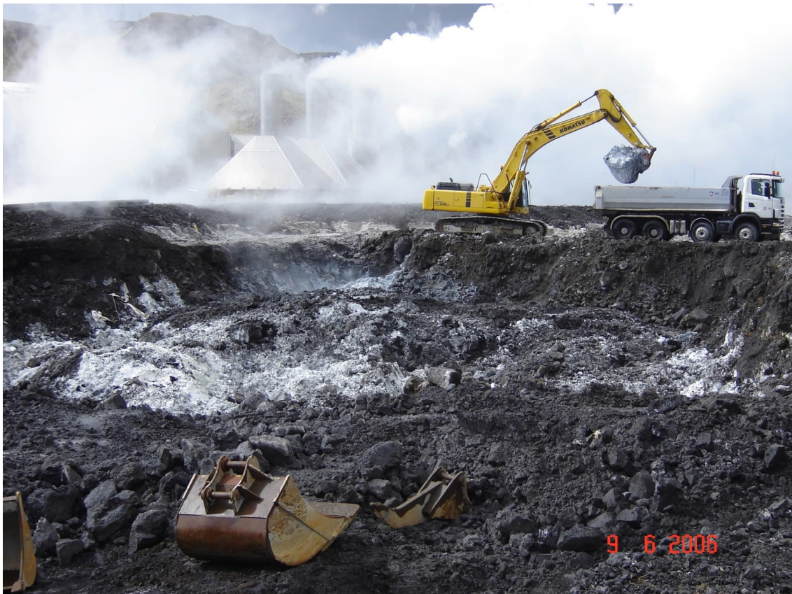
Figure 3.1 Power station 6 under construction June 2006.
